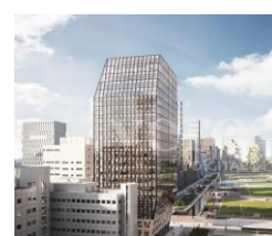
NSI –Well House - Bureaux Amsterdam 24 000 m 2
